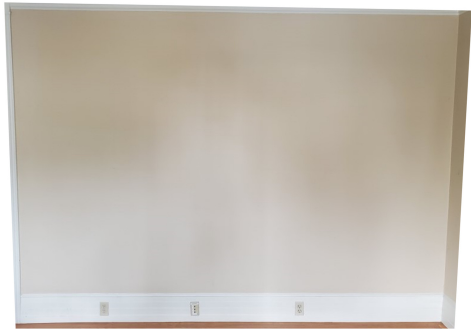
Figure 4. The wall used for investigating Kinect v2 and Azure Kinect sensor accuracy in horizontal and vertical directions.
